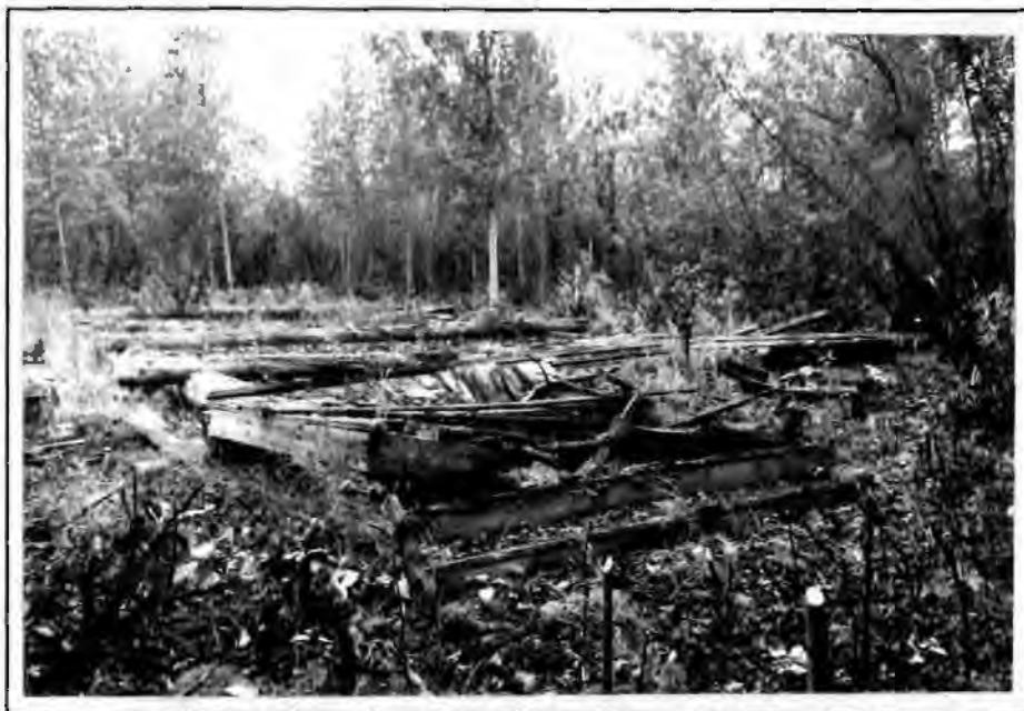
Figure 106. The ruins of the Wadsworth House, 1993. The view is looking west.
